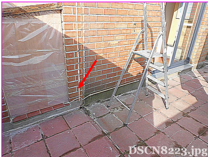
Loshangede bedrading.
